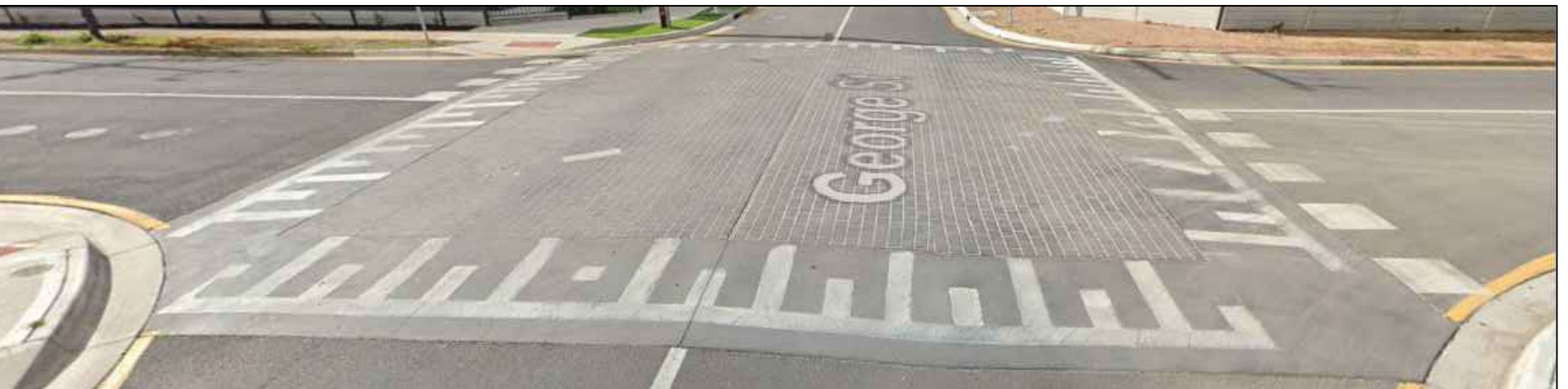
RAISED PAVEMENT AT CROSS INTERSECTION
