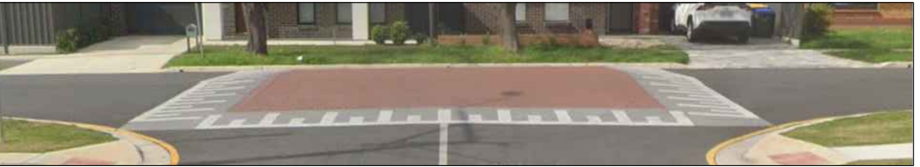
RAISED PAVEMENT AT T-INTERSECTION
