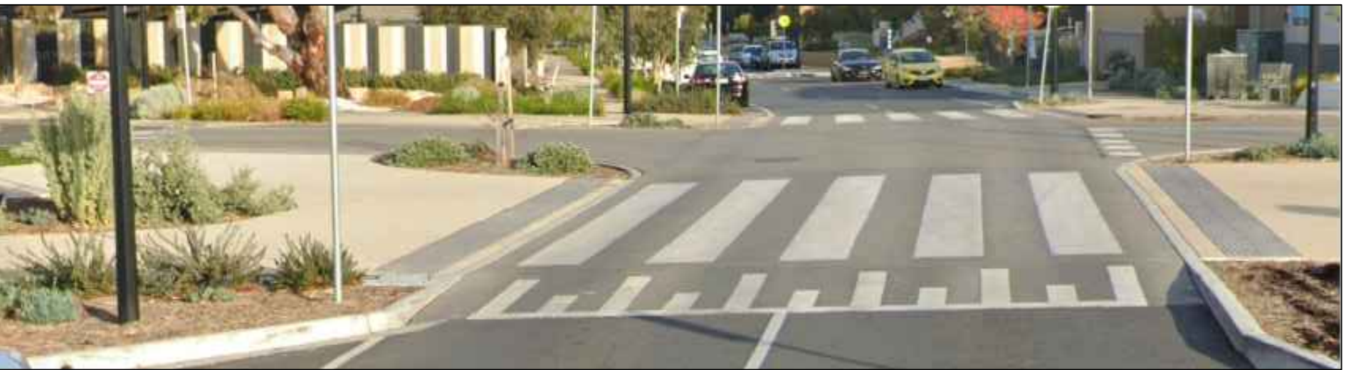
RAISED INTERSECTION WITH PEDESTRIAN FACILITY
