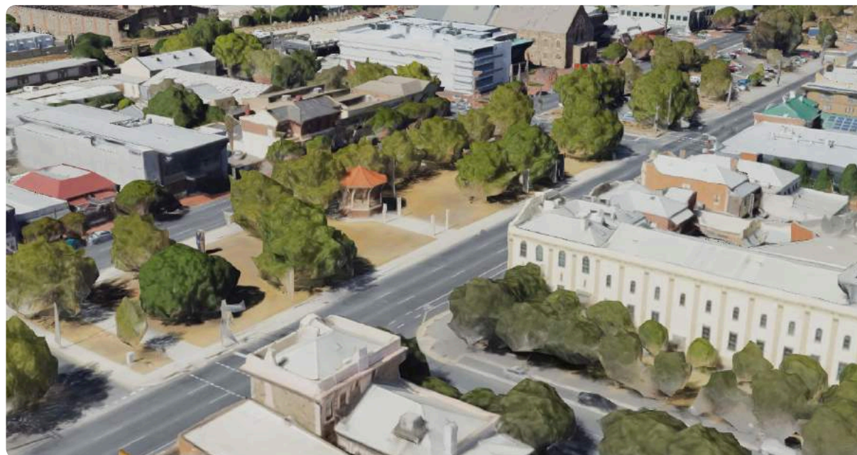
Figure 6 Above left: A daytime view of the Hindmarsh Bandstand at Chief St. Right: The historic gas lamps lit up at night. Below: The gateway improvement focus area encompassing the Hindmarsh Bandstand and gas lamps on Port Road.
