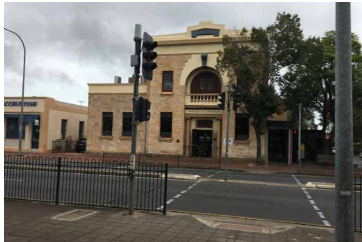
NNQ building and crossing
