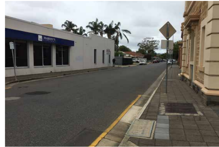
Kemp St verge condition
