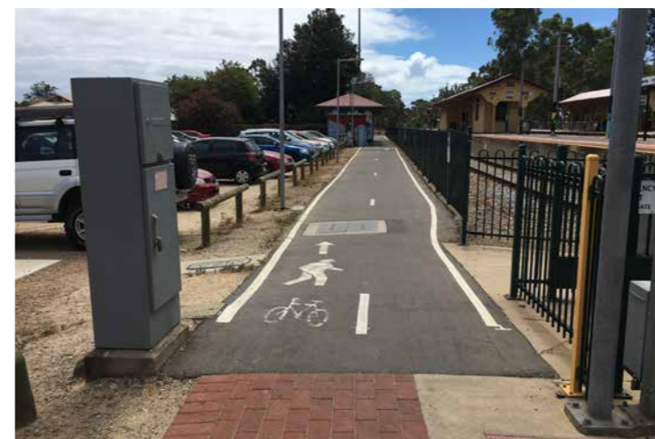
Woodville Station with shared path
