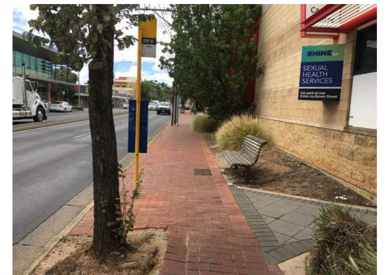
Narrow verges with constricted footpaths and minimal public transport facilities.
