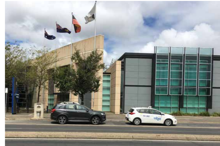
Civic Centre and forecourt
