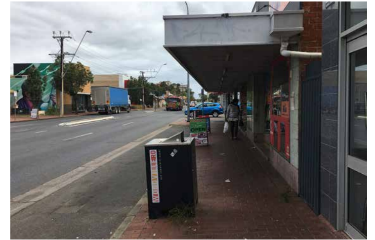
Woodville Rd verge condition
