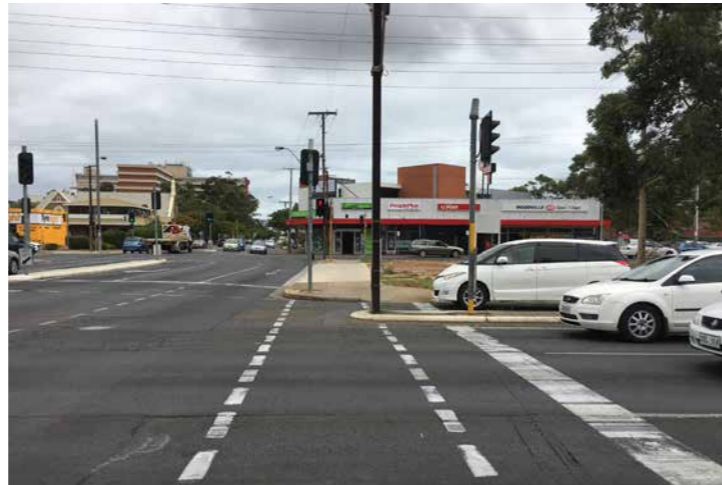
Port Road/ Woodville Road intersection
